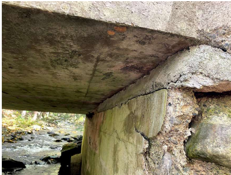
Significant Spalling
