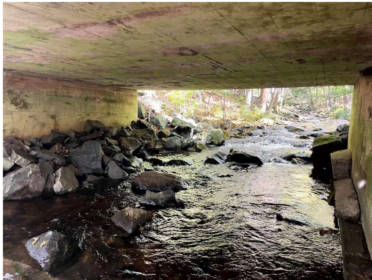
Underside of Deck in Good Condition
