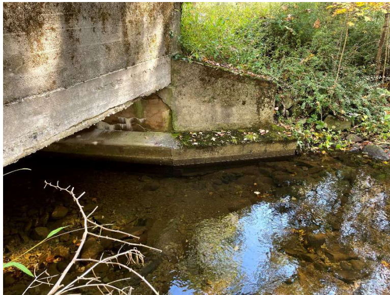
Downstream w/ Wing Wall
