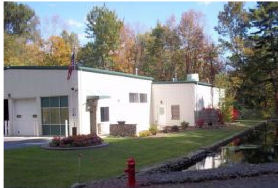
Fig. 4.3, Water Authority Building, www.milfordpawater.com
