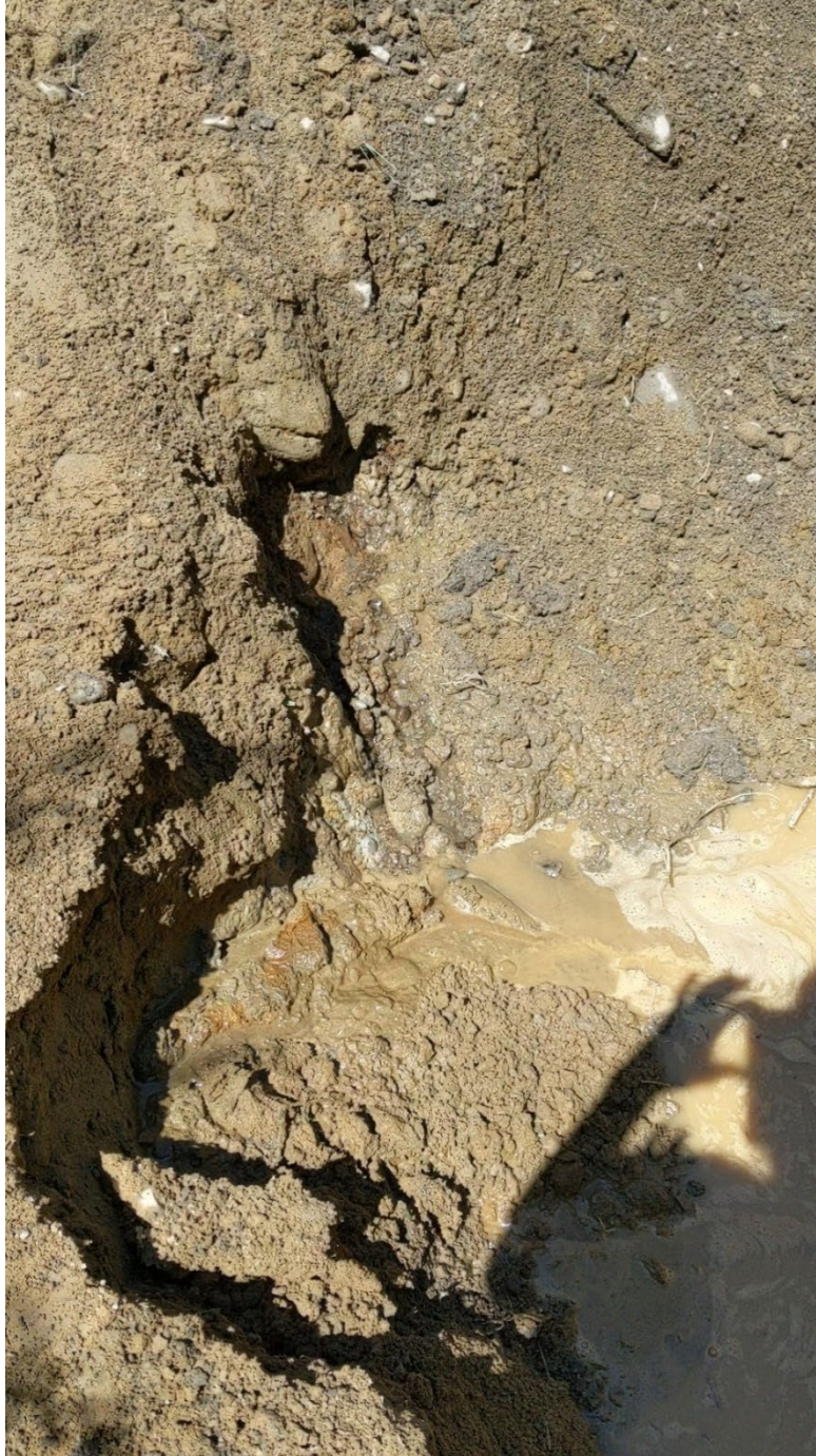
I-6E Water enters from pebble and cobble layer on west side at bottom. Sand, pebbles, and cobbles in west wall of excavation
